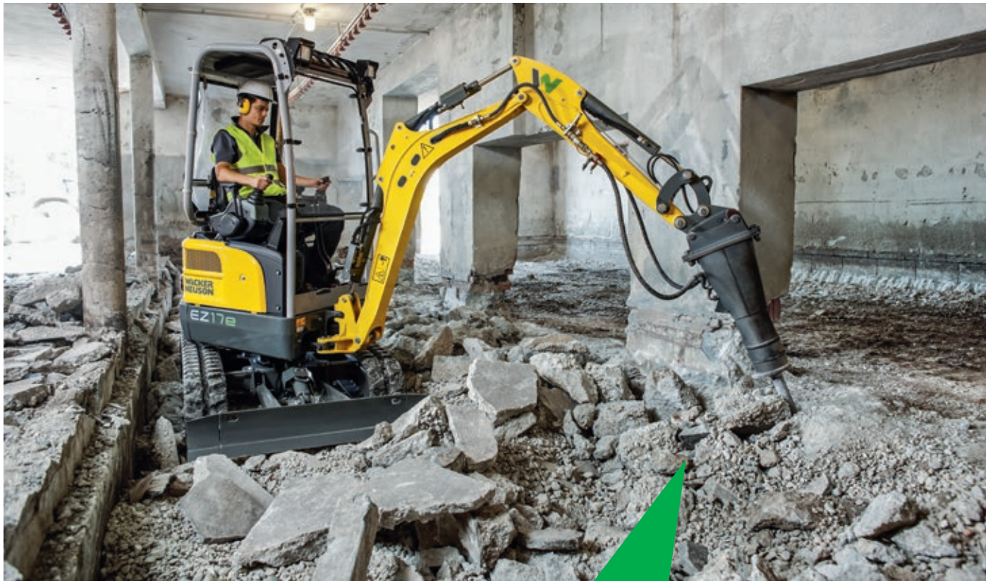
Typical application: indoor spaces Safe deployment indoors: the electric excavator EZ17e
