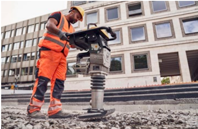
The battery-powered rammers save on noise and emissions, particularly in inner-city construction sites, and as a result, protect the construction site environment.
