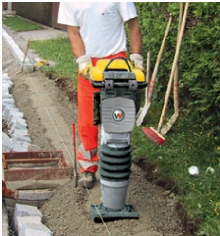
Exact unit guiding - important during compaction in border areas.
