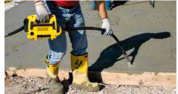
**Economical solution:** with a modular system for optimally compacted concrete with the Basic line HMS.
